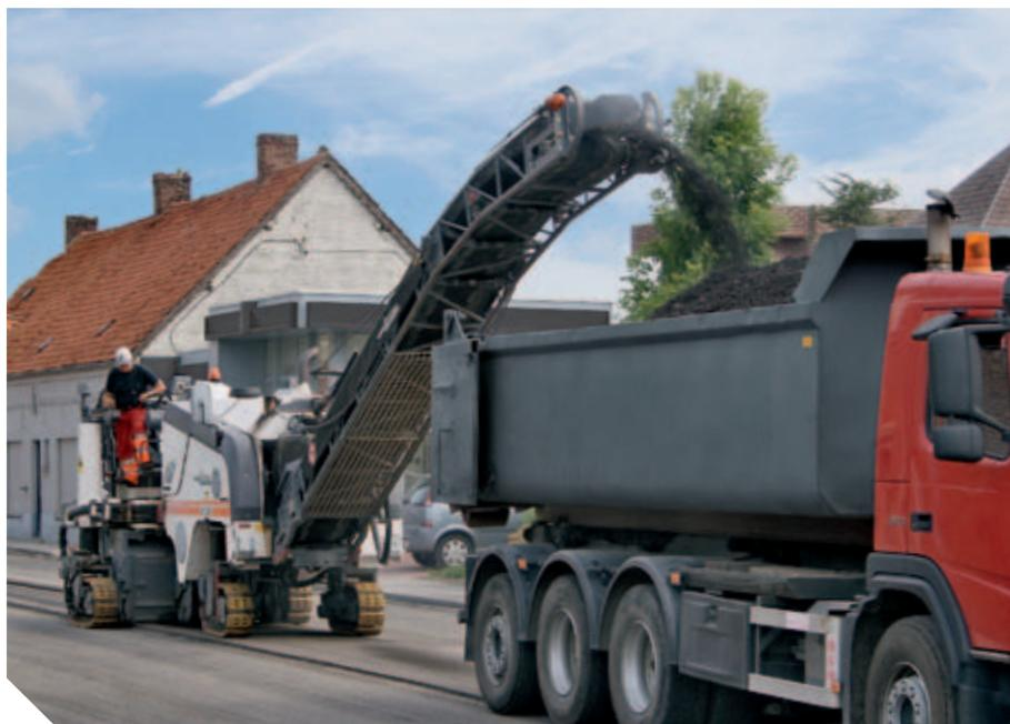
▲ The gradation control beam is pressed down hydraulically to produce small-sized material and prevent the pavement from breaking into slabs
